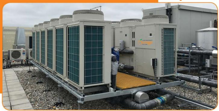
These Air Sourced Heat Pump's uses natural source of heat air to produce energy. They absorbs warmth from the outside air and converted it into heat. This Heat Pump working on principle of vapour compression refrigeration, an Air Sourced heat pump uses refrigerant system involving compressor and condessor to absorb heat at one place and release it at another place.
